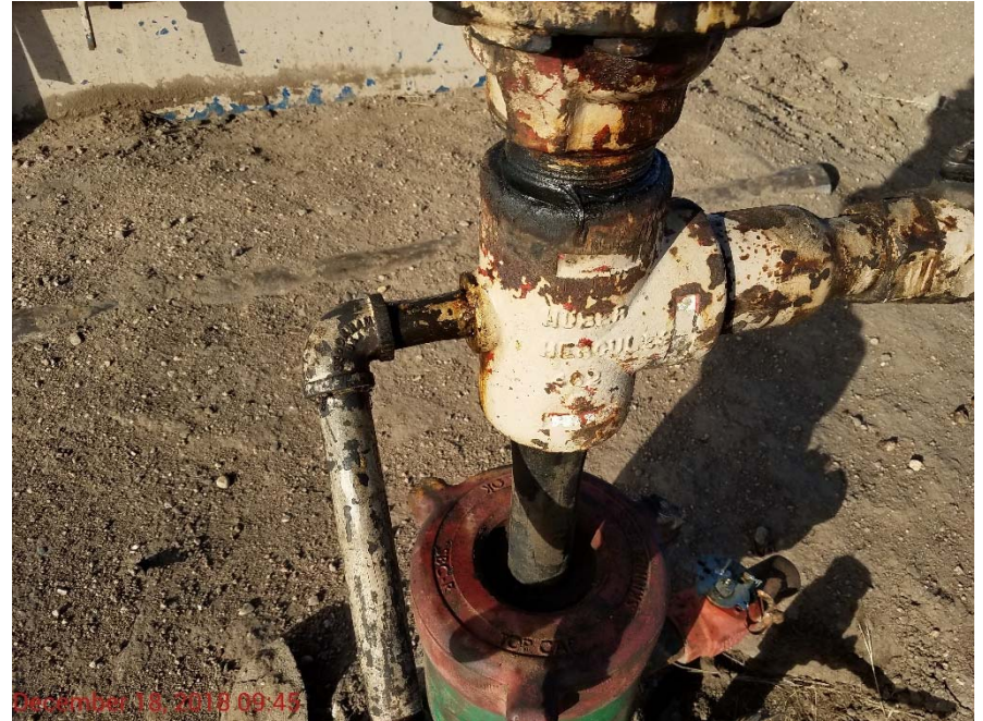
Photo 4 – Leaky fitting at Federal North Wildhorse 7-28 wellhead. Operator contacted via phone to repair gas leak.
