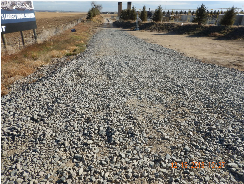
Photo 11. Photo taken from the entrance of the location, facing East. Vehicle tracking BMP appears to be in proper functioning condition.
