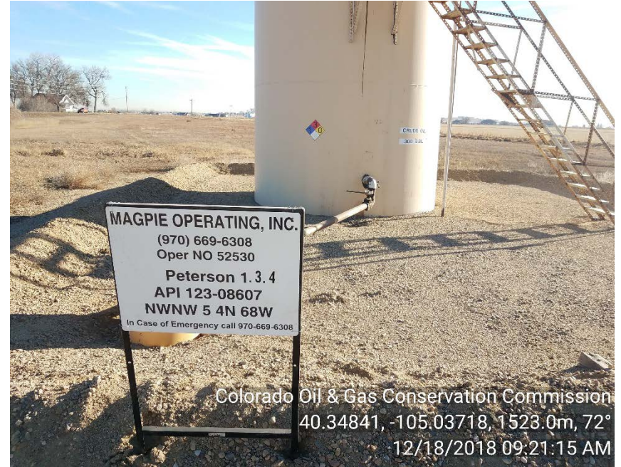
Crude oil tank and battery sign on 12/18/18
