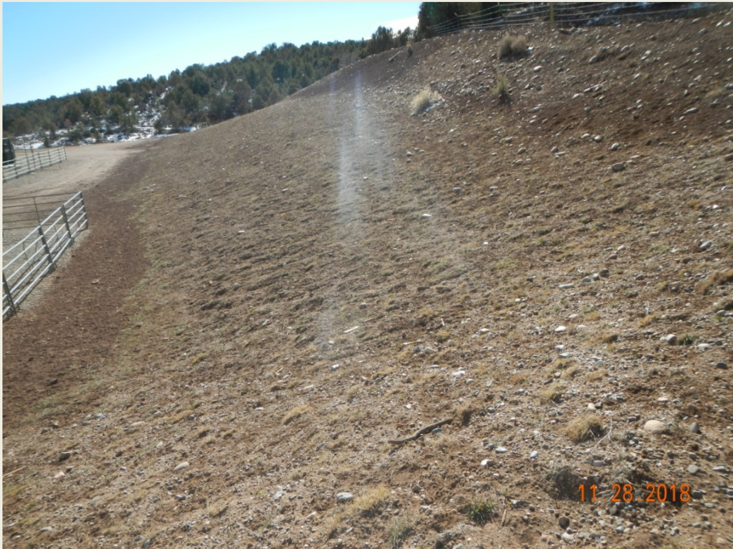
Photo 2. View of the western project area from the northwestern corner facing southward. Revegetation is sparse and appears grazed. This needs to be monitored and revegetation installed if erosion worsens. Cattle exclusion may be needed.
