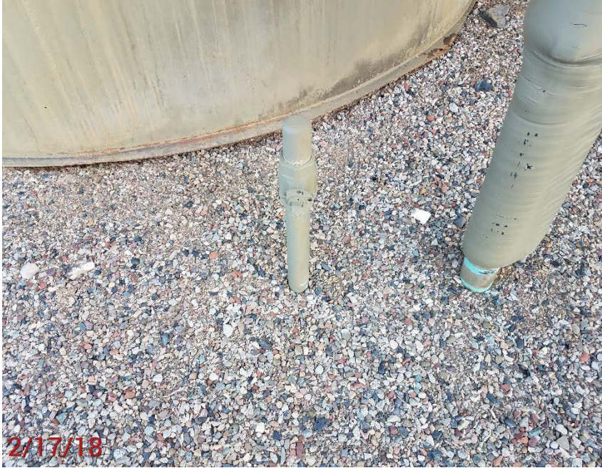
Location Photo #5, Unmarked flow line riser in tank battery.
