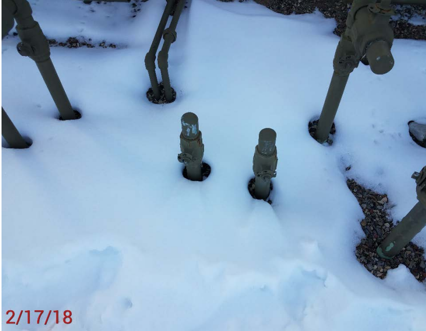
Location Photo #3, 2 Unmarked flow line riser at separators.
