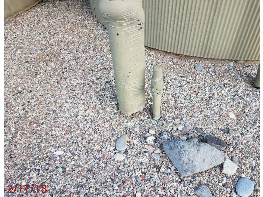
Location Photo #4, Unmarked flow line riser in tank battery.
