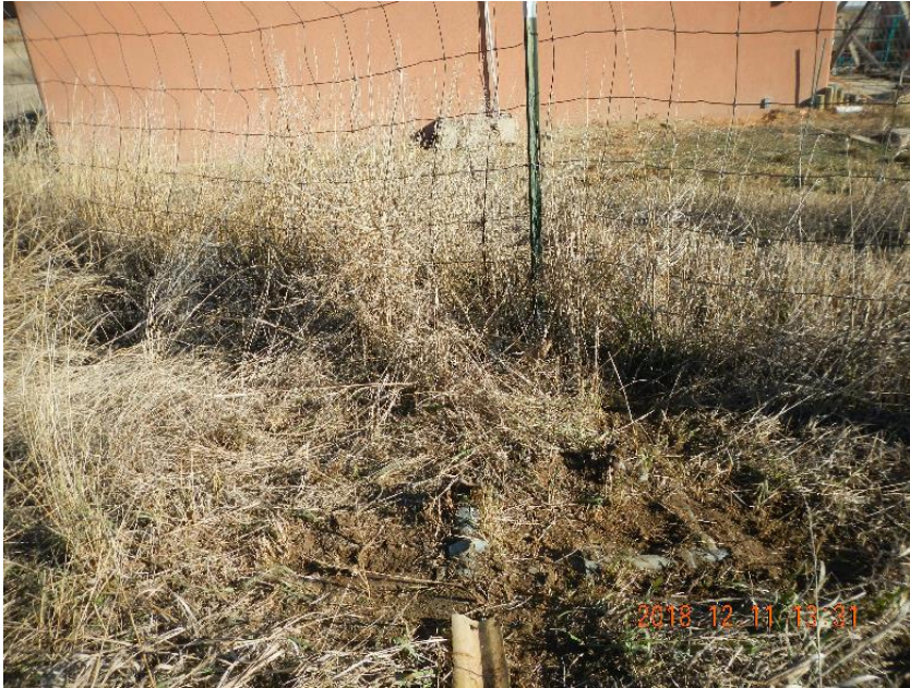
Photo 3: 1" flowline at elbow and valves turning E to residence.
