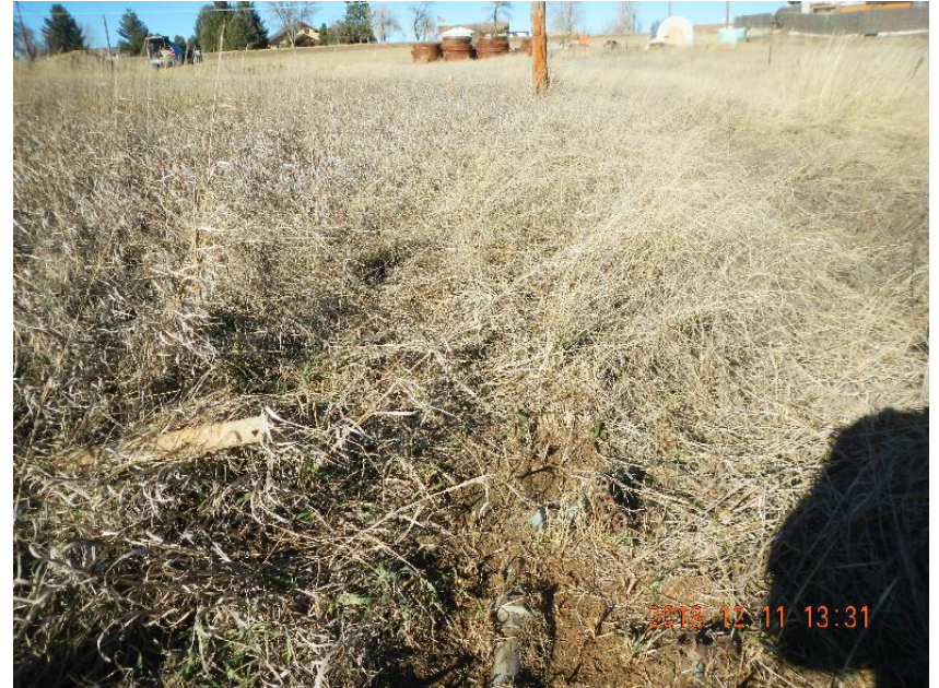
Photo 2: 1" steel line on W side of fencing looking NE towards wellhead.
