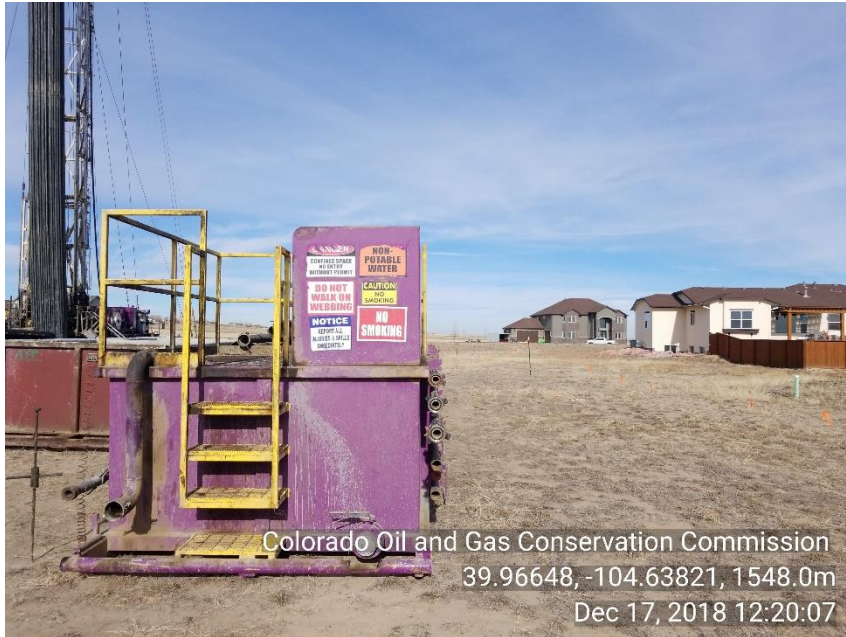
Photo 3 Work over rig to house
