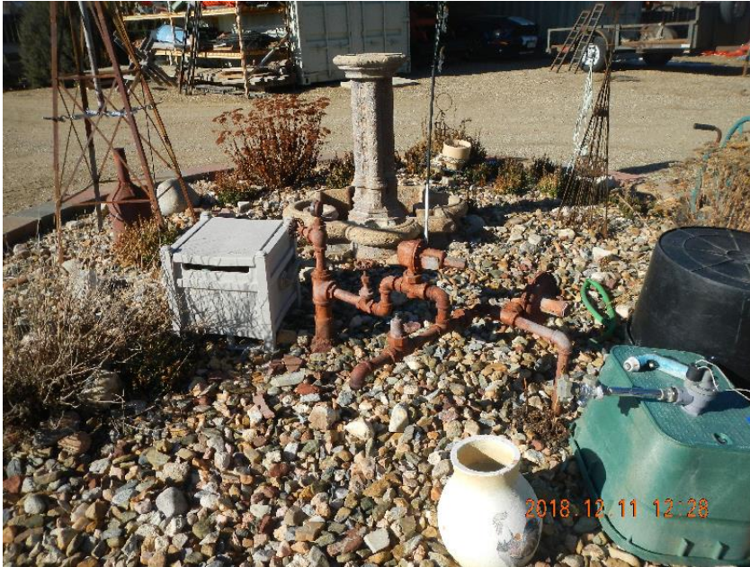
Photo 1: Wellhead and flowline with steel riser back and to the left of wellhead.
