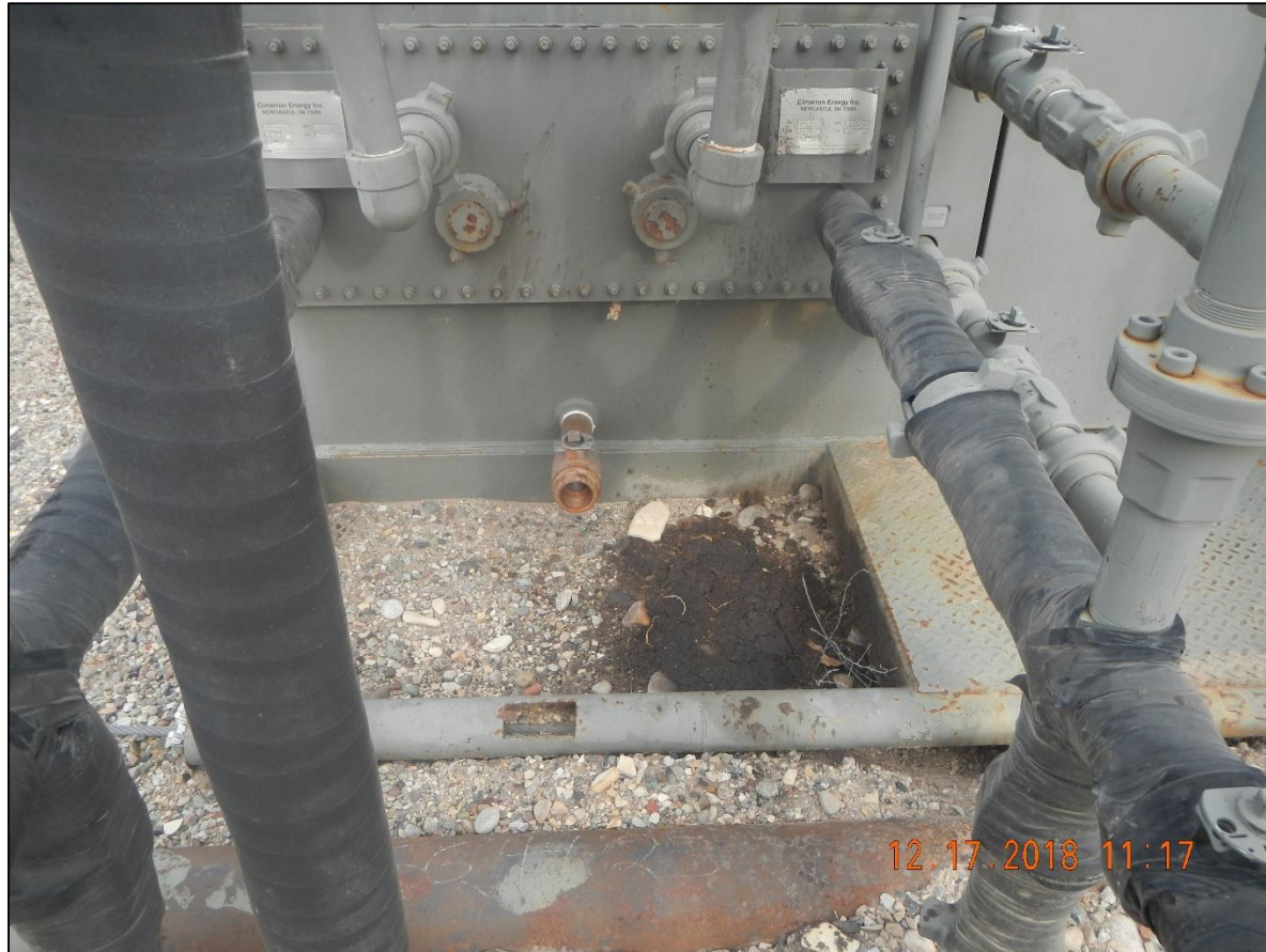
Stained groud in front of separator (SG 333-23/SG 433-23)
