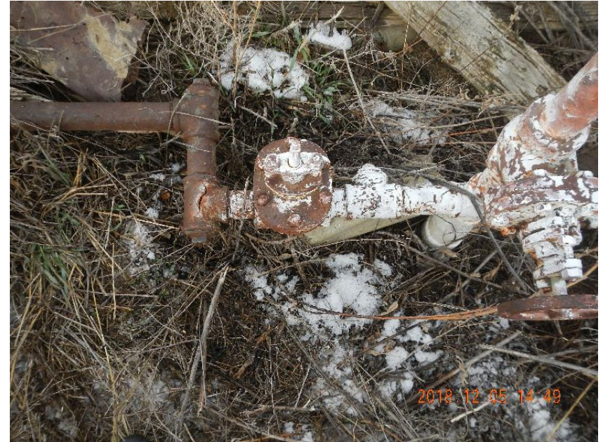
Photo 2: Flowline off W side of wellhead with split in T.
