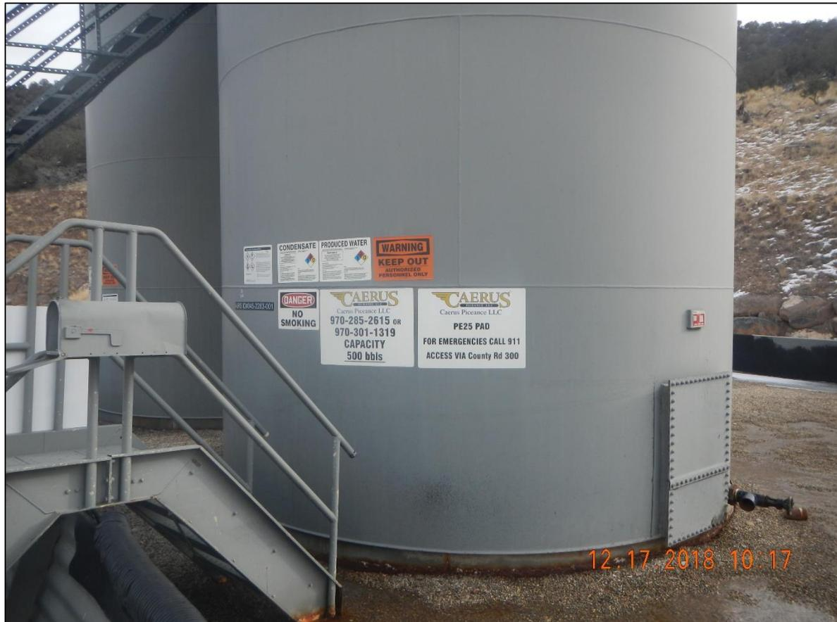
**The phone number for local emergency services (911 where available) and the public road used to access the site is on a label on production tank in tank battery.**
