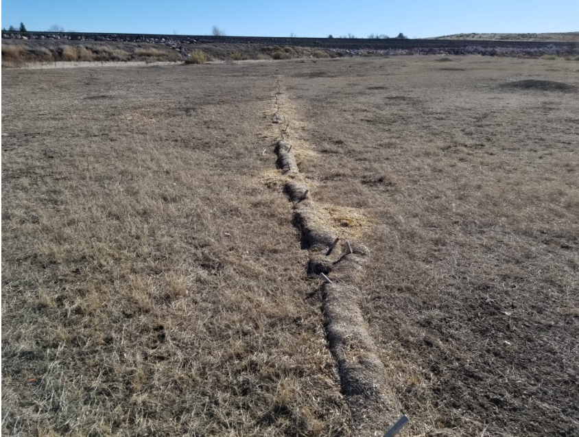
Photo 3. Photo taken from the location, facing South. Erosion control waddles left on site are deteriorating.
