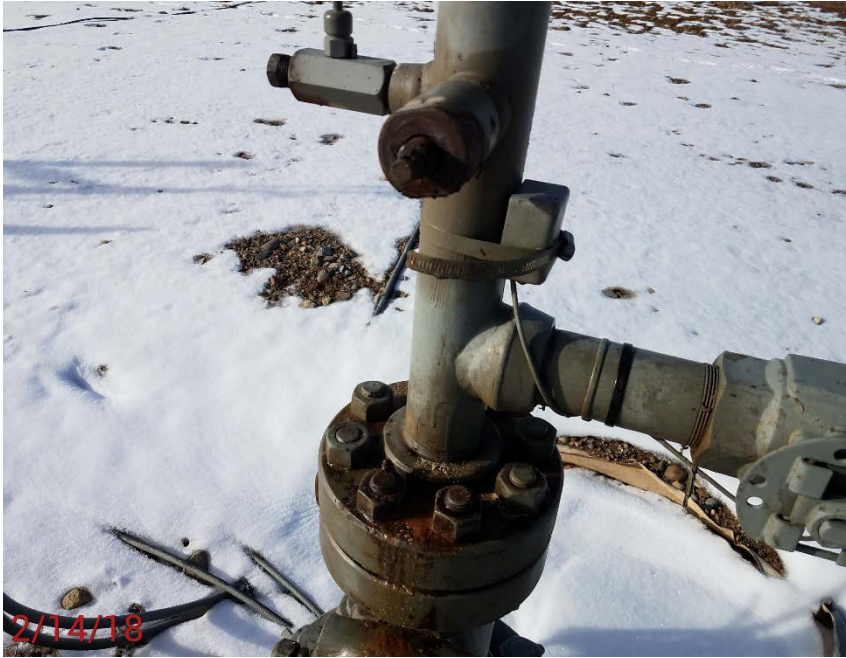
Location Photo #3, Leaking plunger catch on well 36-10
