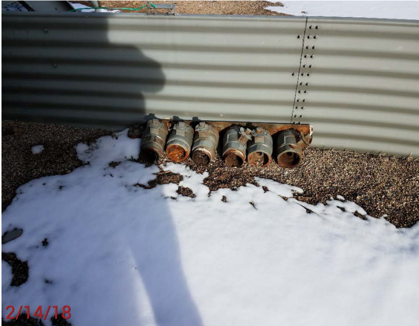
Location Photo #5, Unused valves in battery.
