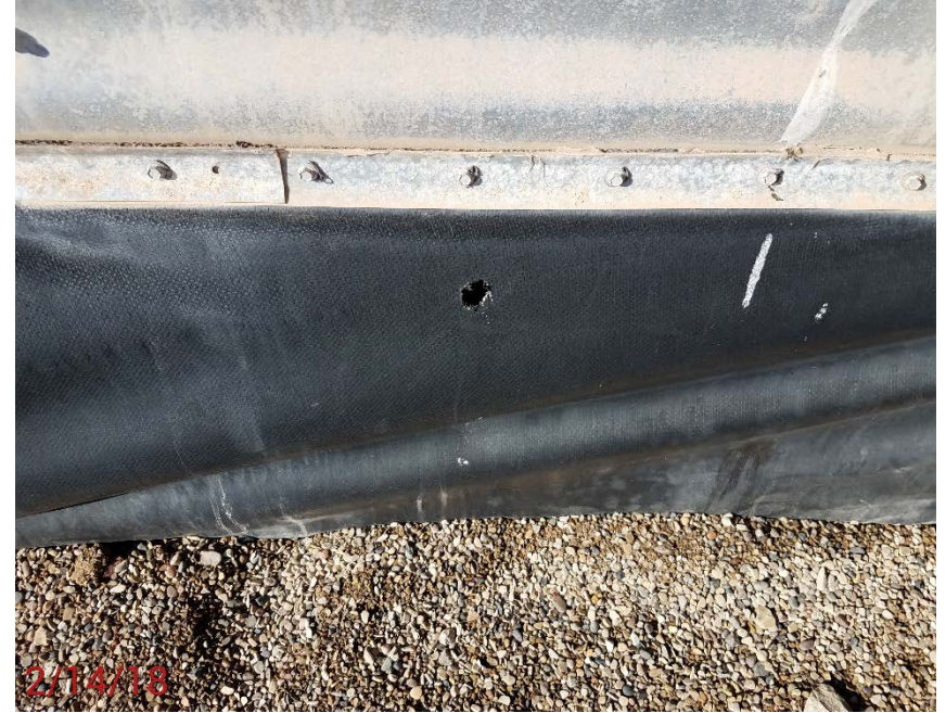
Location Photo #4, Several holes in battery containment liner.
