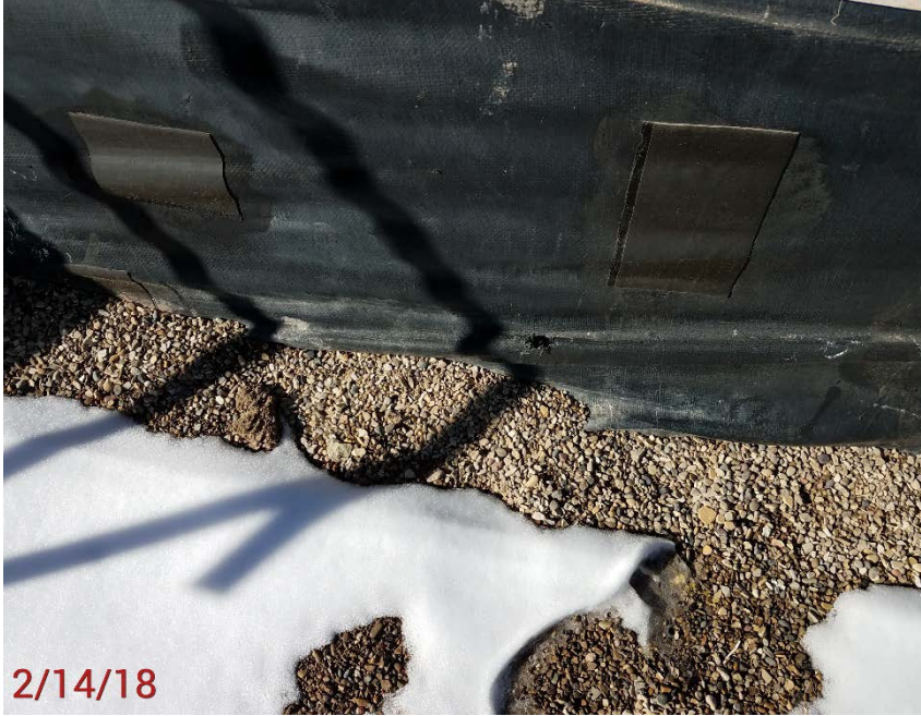
Location Photo #3, Several holes in battery containment liner.
