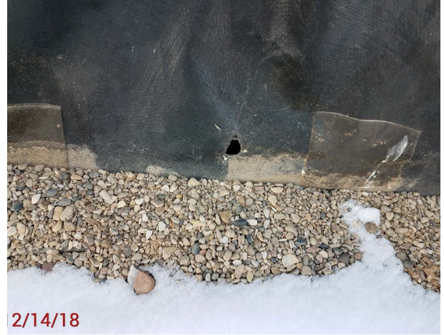
Location Photo #6, Several holes in battery containment liner.
