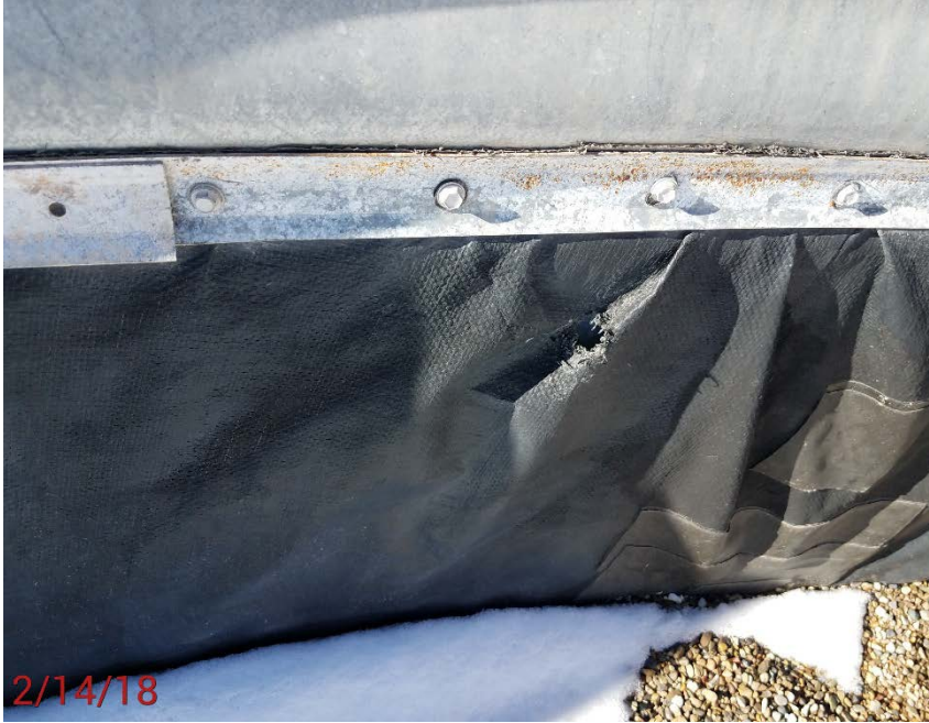
Location Photo #5, Several holes in battery containment liner.
