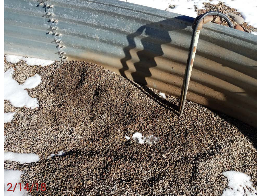
Location Photo #6, Oil stained rock in battery containment.
