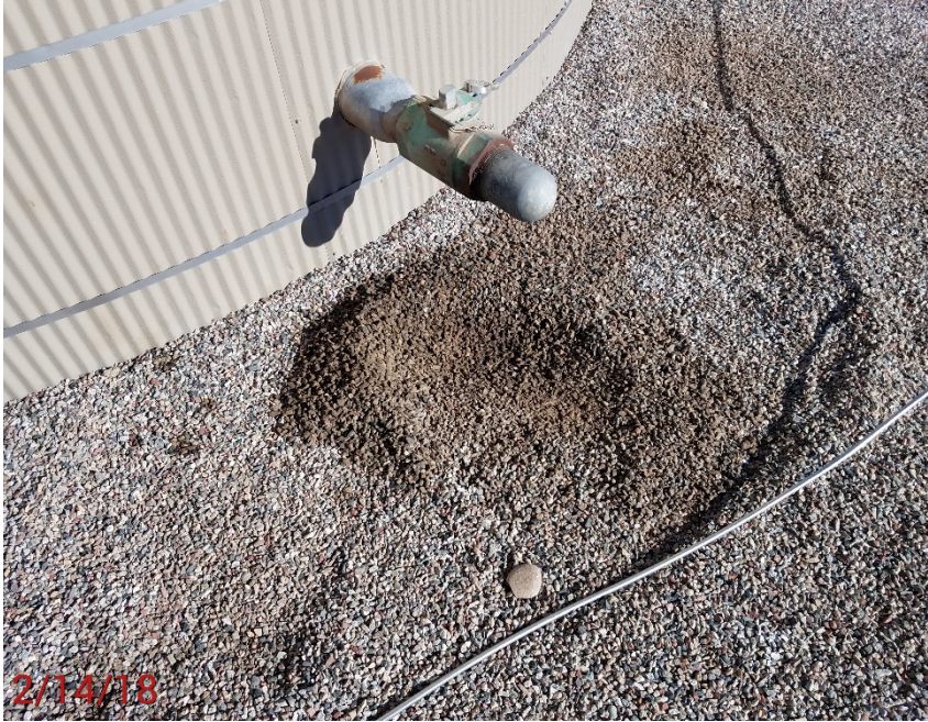
Location Photo #5, Oil stained rock in battery containment.
