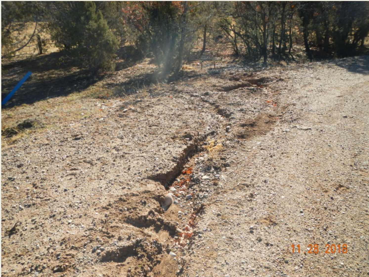
Photo 5. View of erosional channel at the entrance to the well pad measuring approximately 12 inches wide and deep.
