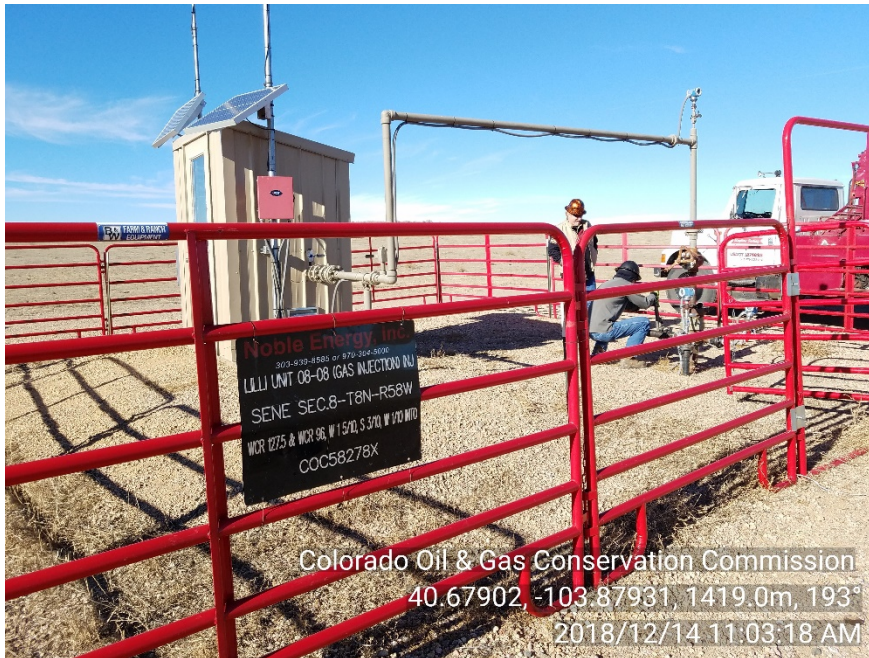
Photo #1 Lilli Unit 8-8 (API 05-123-13862) Wellsite sign – UIC-MIT
