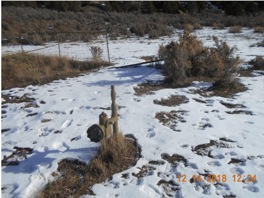
Meter housing removed. Flowline riser blinded.
