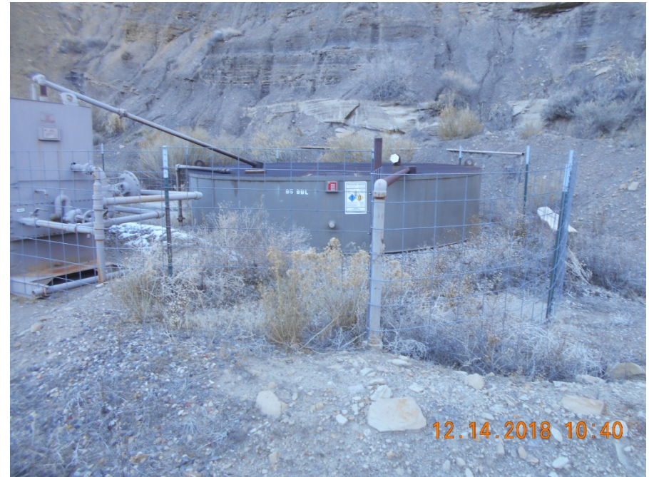
95 bbl blowdown tank with fence
