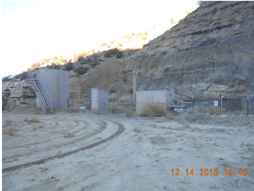
Separator , Meter housing, Tank battery
