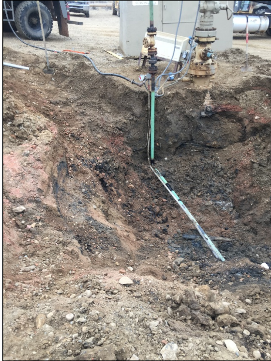
Steel Flowline from injection pump to wellhead
