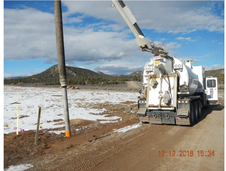
Hydro vac truck preparing to expose pipelines along western edge of roadway.
