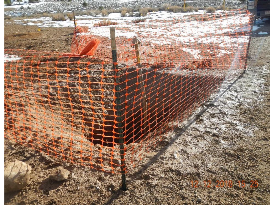
Hydro vac excavation to expose pipeline along eastern edge of access road.
