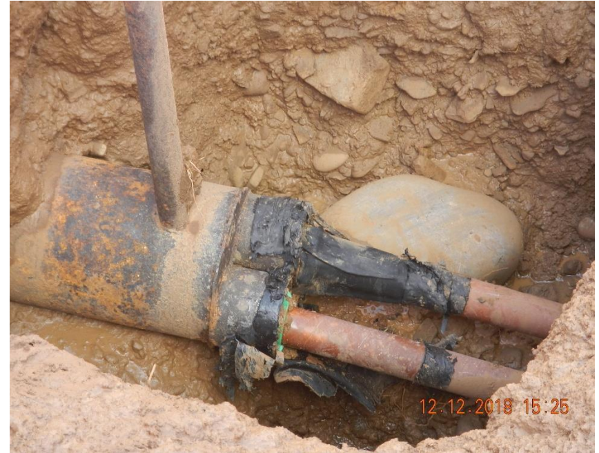
Exposed 3" fiberglass pipelines within 12" casing sleeve.
