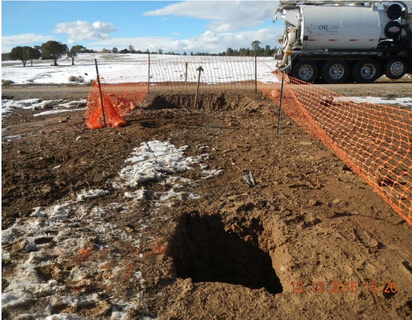
Potholed Williams pipeline in foreground.
