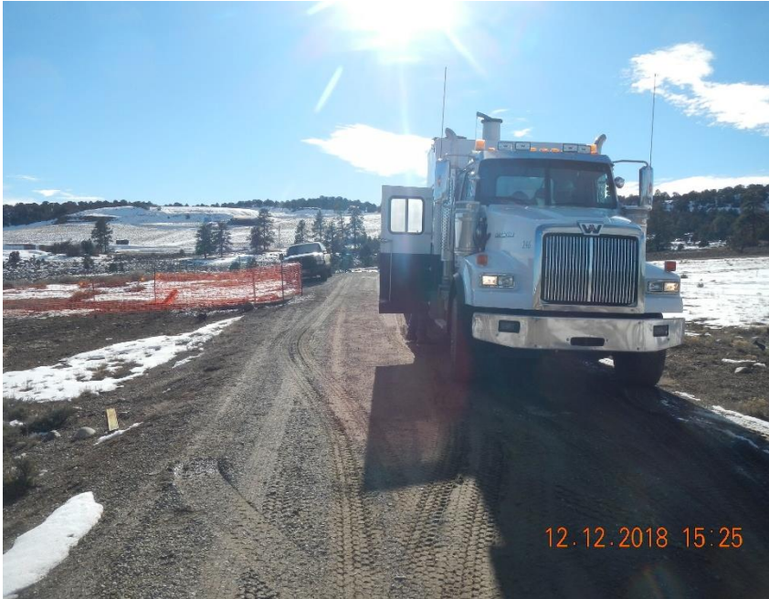
Vac truck preparing to expose pipeline along western edge of access road.
