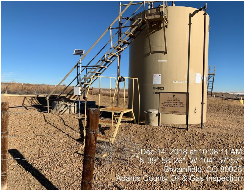
Photo#1 Produced Oil Tank and Produced Water Pit
