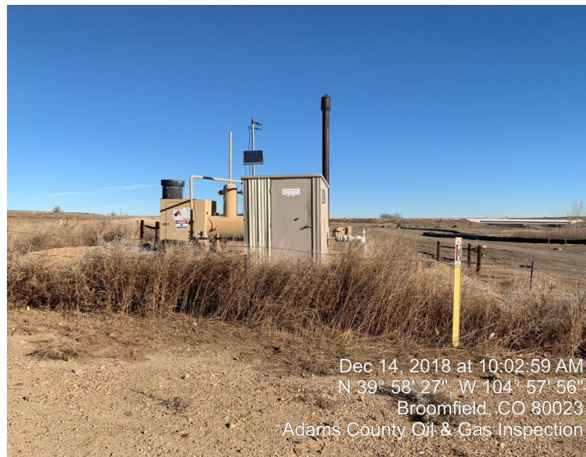
Photo#2 Gas meter/Separator/ECD
