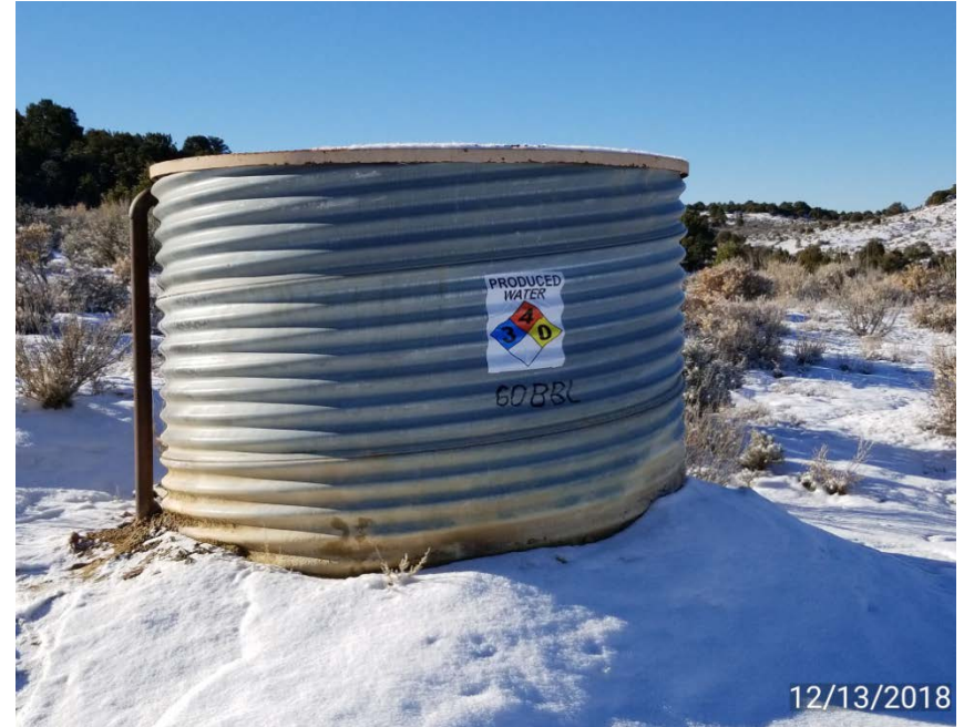
Photo 2. 60 bbl labeled water tank without berm.
