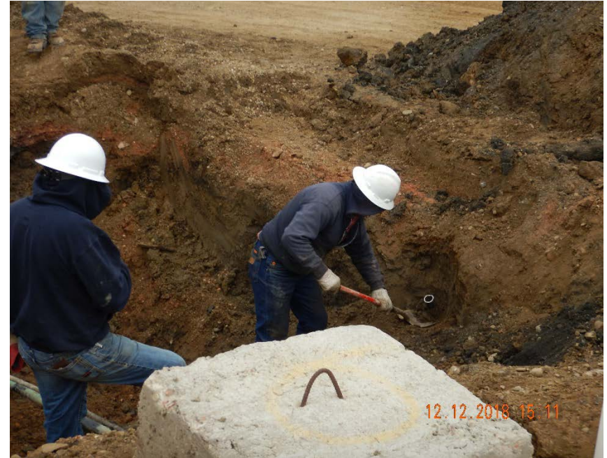
Photo #6 – Operator was instructed by COGCC Western Integrity Supervisor to cap unidentified 2" flowline that was exposed on east side of excavation.
