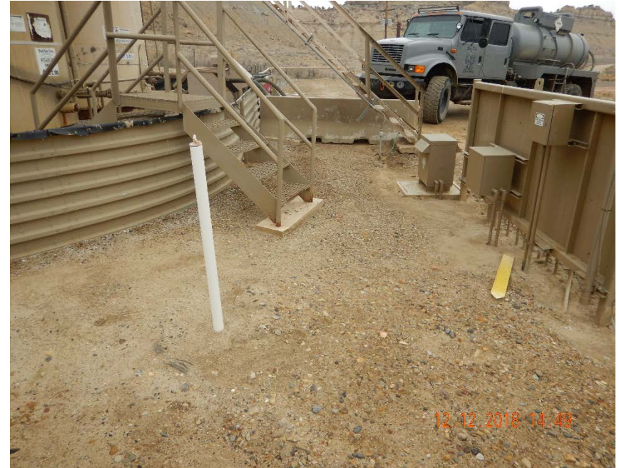
Photo #4 – Additional PVC riser (monitoring well) located between excavation and tank battery.
