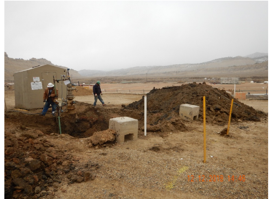
Photo #2 - View of additional excavated soil stockpile east of excavation. Note two capped PVC risers (monitoring wells) located south of excavation and east of stockpile.
