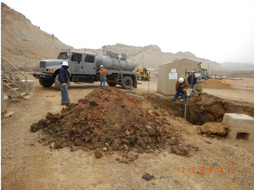
Photo #1 – Overview of flowline integrity test configuration from south of excavation. Note stockpile of excavated material in foreground.
