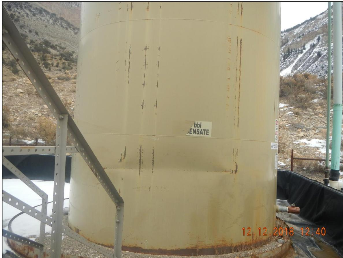
Capacity label is torn off of tank.
