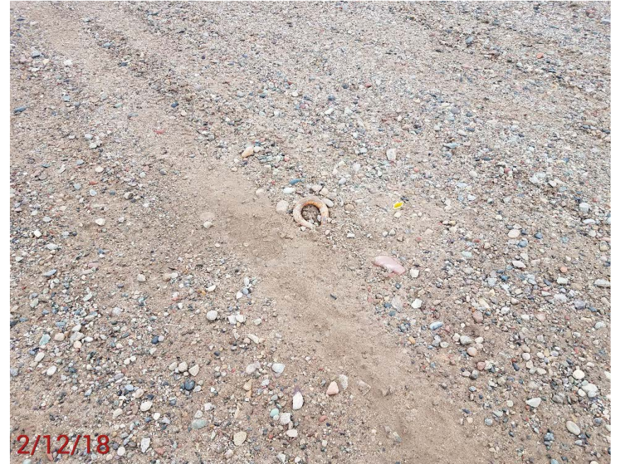
Location Photo #8, Unmarked deadman anchors.
