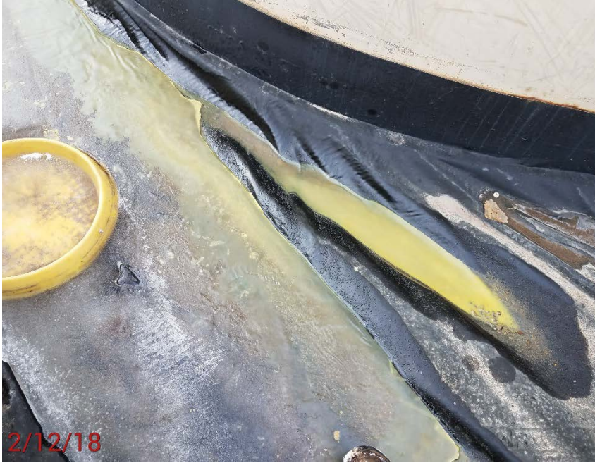
Location Photo #4, Spilled condensate in battery containment.
