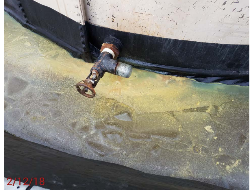
Location Photo #5, spilled condensate in battery containment.
