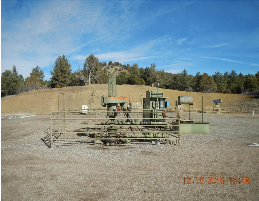
Burkett A #2 location photo.
