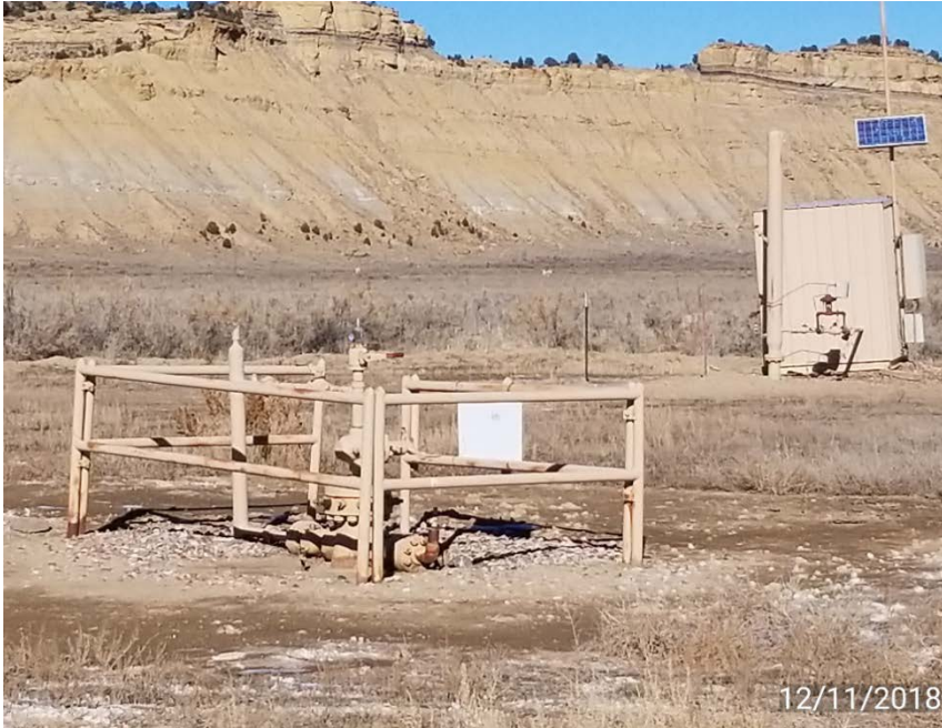
Photo 1. Location looking northwest.
