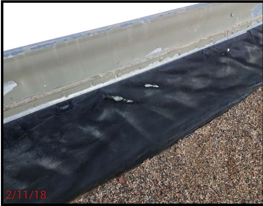
Location Photo #7, Holes in secondary containment liner.
