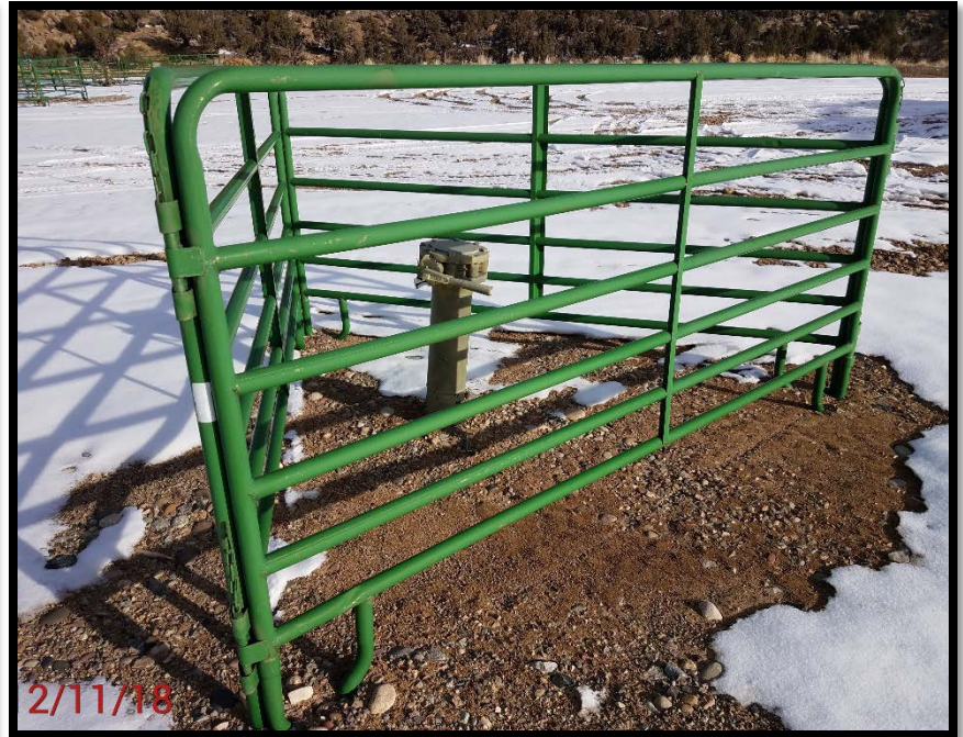
Location Photo #4, unmarked, unused 6" poly riser.
