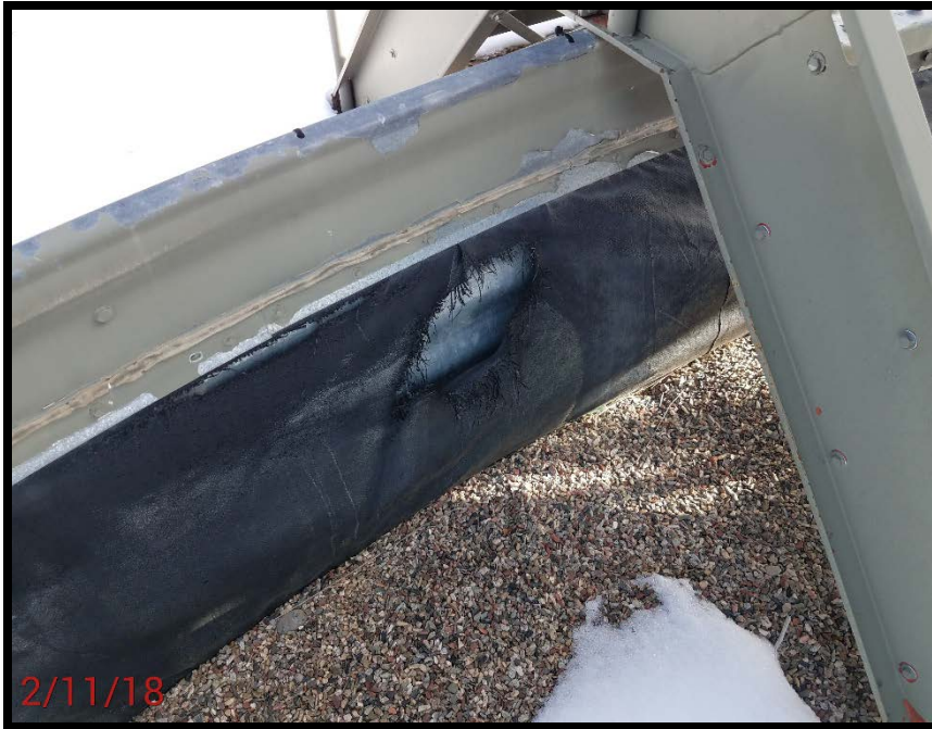
Location Photo #5, Holes in secondary containment liner.
