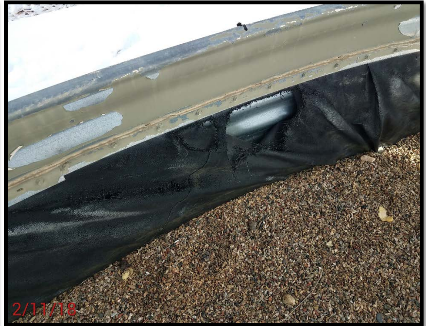
Location Photo #6, Holes in secondary containment liner.
