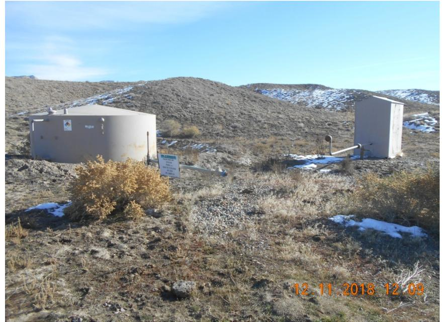
**Tank battery with sign. Meter housing and locked out/tagged out riser.**
