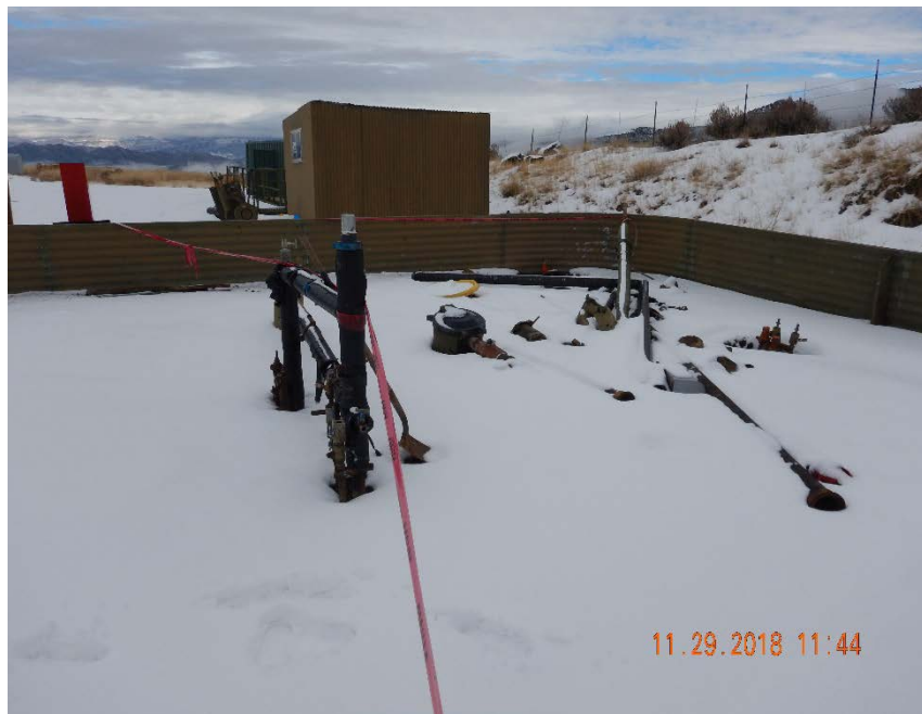
Photo #3 – View of remaining tank battery equipment and flowline risers inside north end of SPCC.
