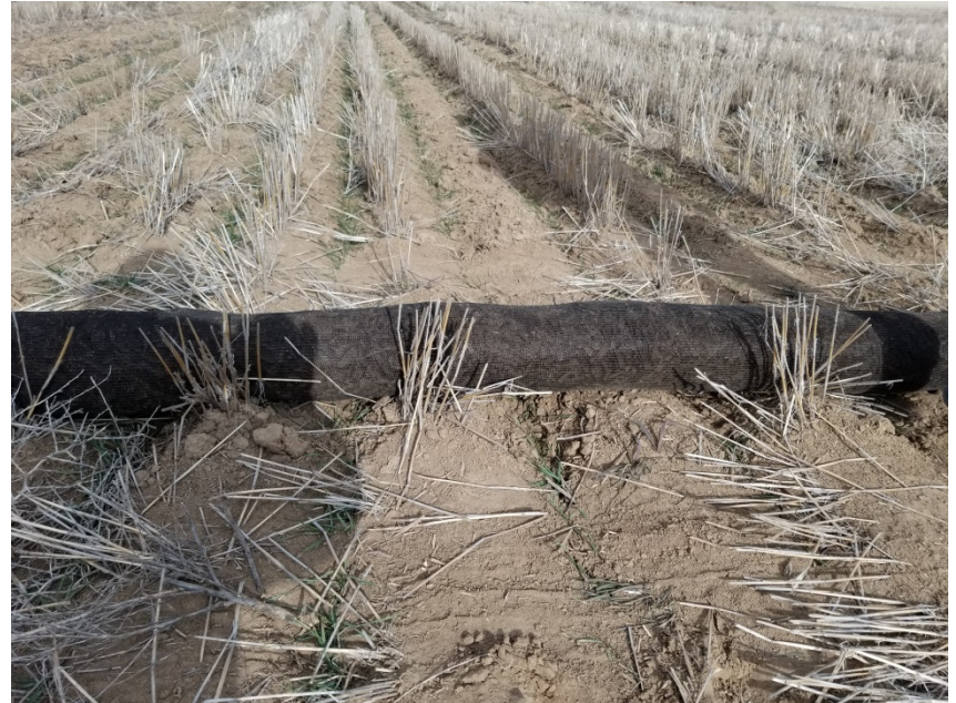
Photo 12. Photo taken from northern perimeter of the location. Photo illustrates filter wattles along the perimeter that need to be trenched in over crop rows due to daylighting underneath.
