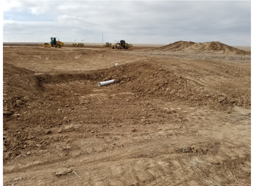
Photo 4. Photo taken from the eastern perimeter of the location, facing East. Operator is in the process of installing a sediment trap with a temporarily stabilized outlet.
