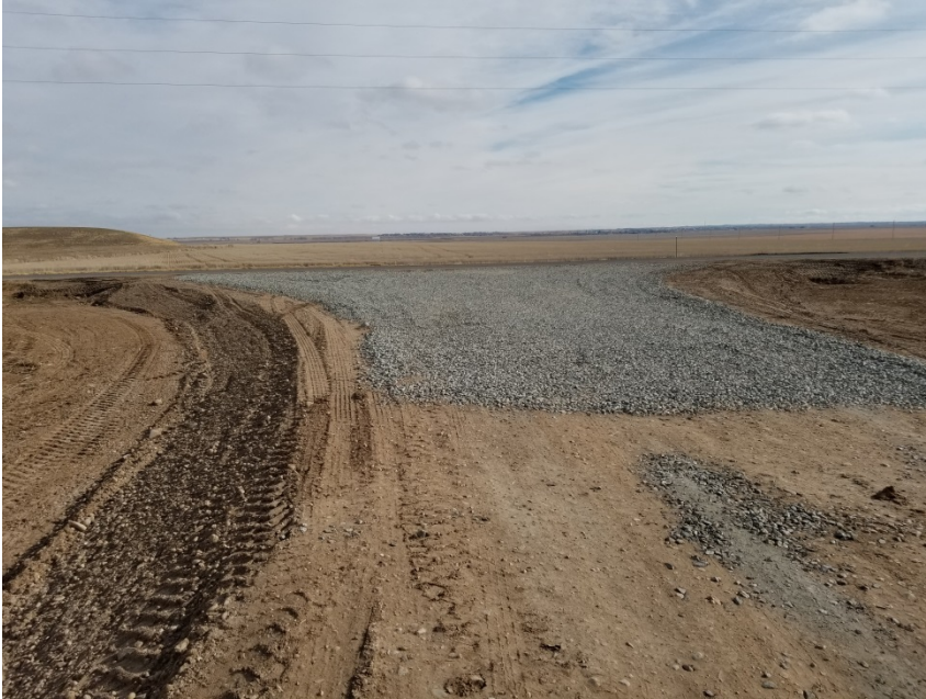
Photo 1. Photo taken from the entrance of the location off CR 21, facing North. Operator has installed vehicle tracking pad. BMPs in proper functioning condition at the time of this inspection.
