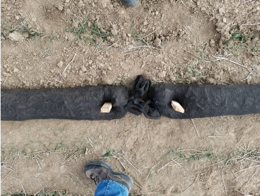
Photo 11. Photo taken from northern perimeter of the location. Photo illustrates filter wattles along the perimeter that need to be overlapped.
