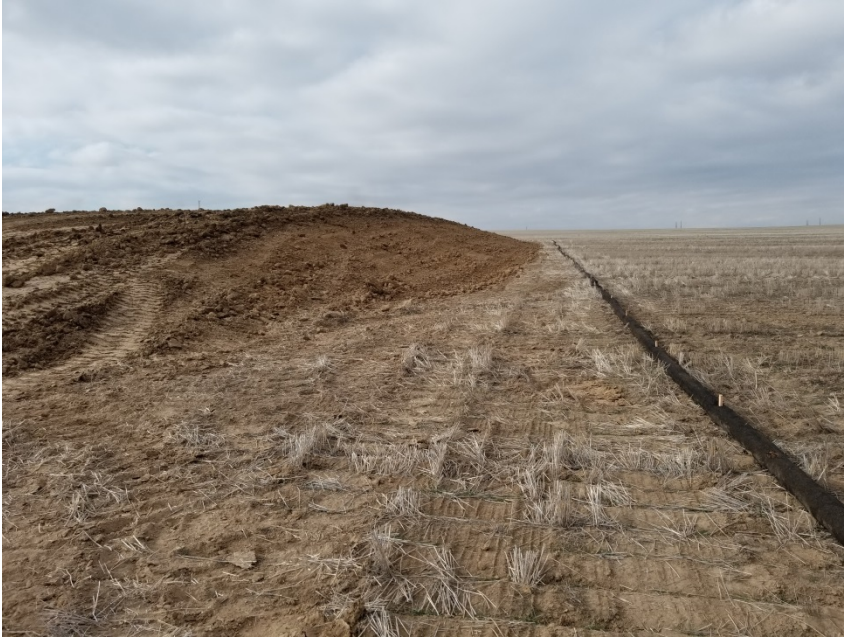
Photo 5. Photo taken from the northeastern perimeter of the location, facing West. Photo illustrates filtrex wattles along the perimeter outside of the ditch and berm. Photo also illustrates the topsoil stockpile being stored along the eastern area and has been temporarily stabilized with equipment tracking. Also See comments under Photo 2.
