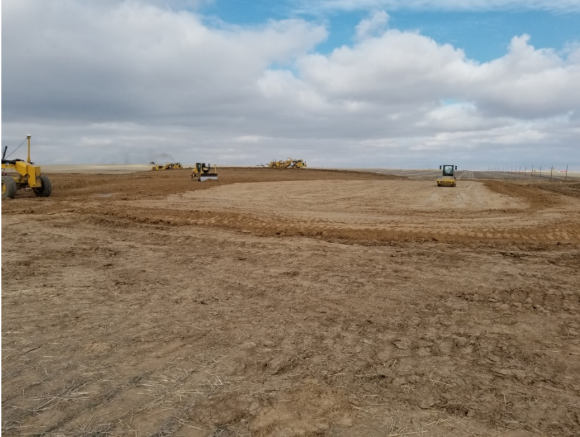
Photo 3. Photo taken from the southeastern perimeter of the location, facing North. Photo illustrates a ditch and berm BMP that has been installed around the entire perimeter of the location in conjunction with other BMPs.
