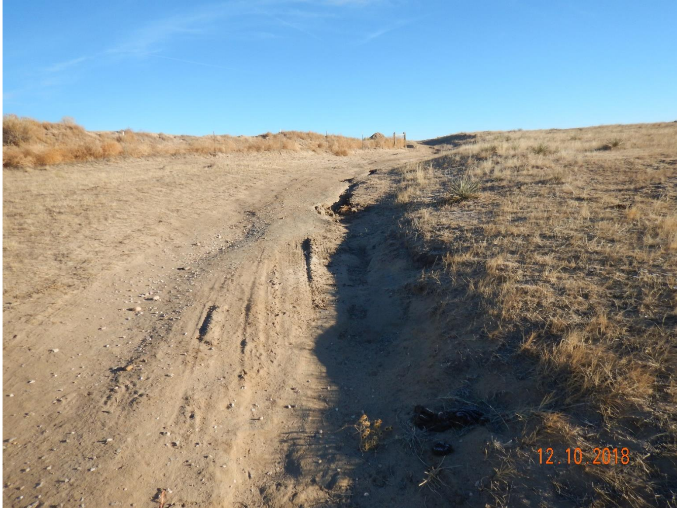
Photo 8: Photo taken from the access road, northeast of the well, facing northeast. Photo shows access road has not been reclaimed, and stormwater erosion degradation has been allowed to continued.
