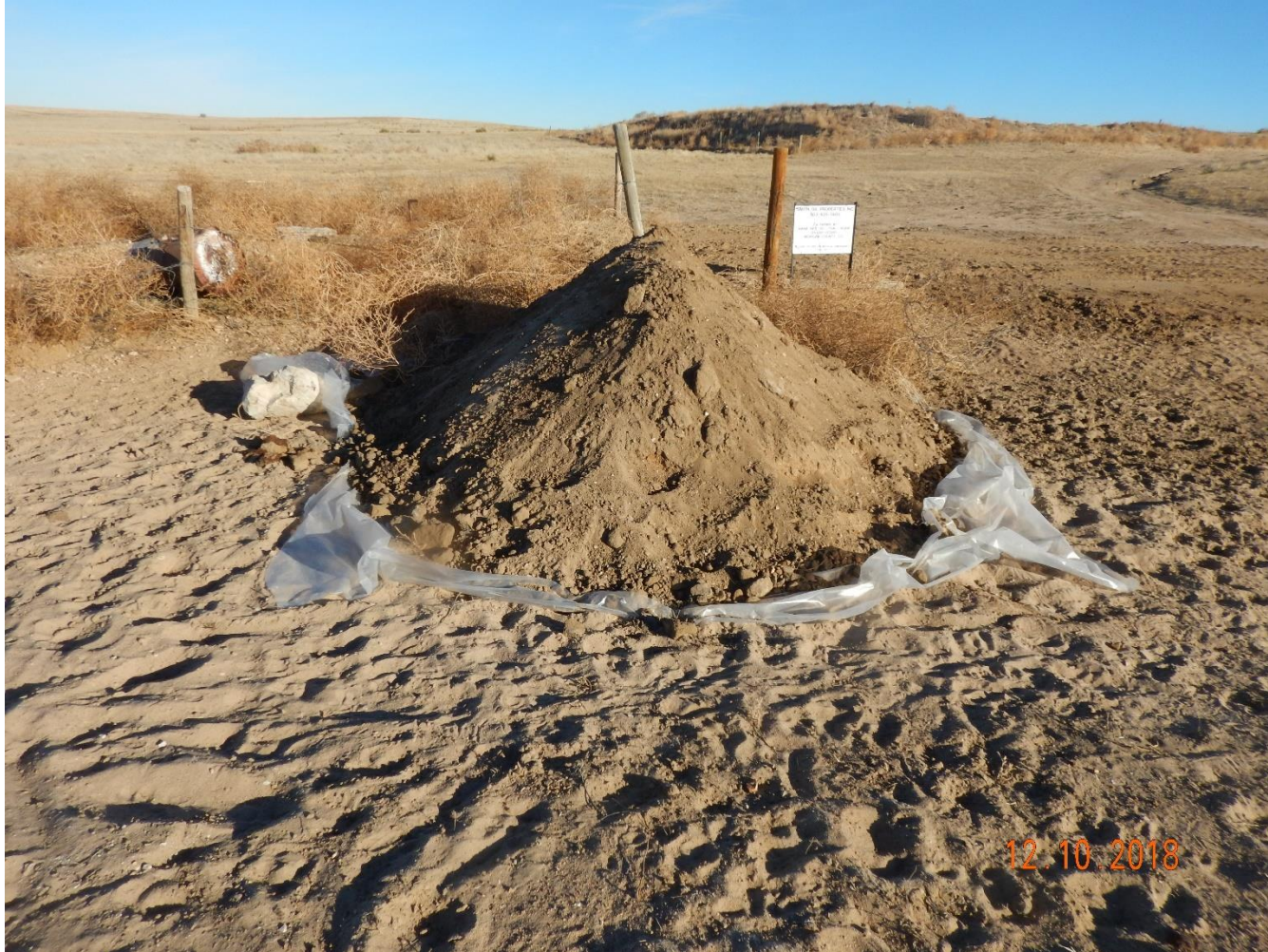
Photo 19: Photo taken from the south end of the well, facing north. Photo shows what appears to be contaminated soil has been stored on the south end of the well with insufficient stormwater and erosion control BMPs
