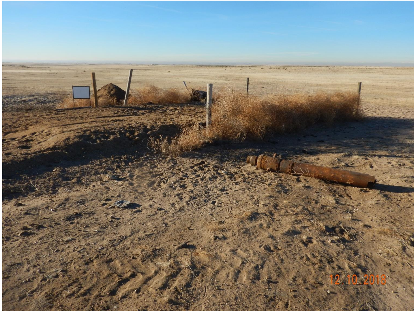
Photo 3: Photo taken from the north end of the well location, facing southwest. Photo shows though pump unit appear to have been removed, no additional reclamation appears to have been conducted in accordance with 1004 rules; various trash debris, equipment and fence remains.
