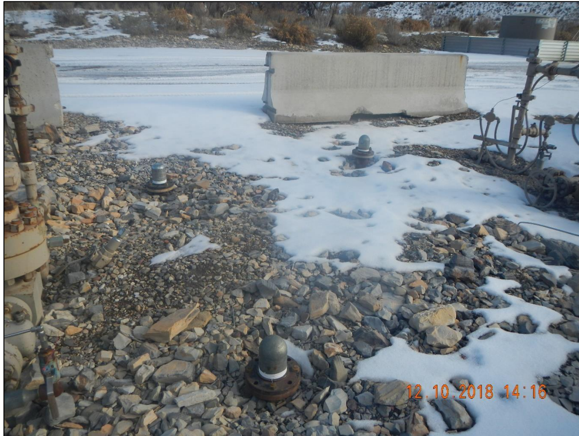
Foundation pipes have been capped.
