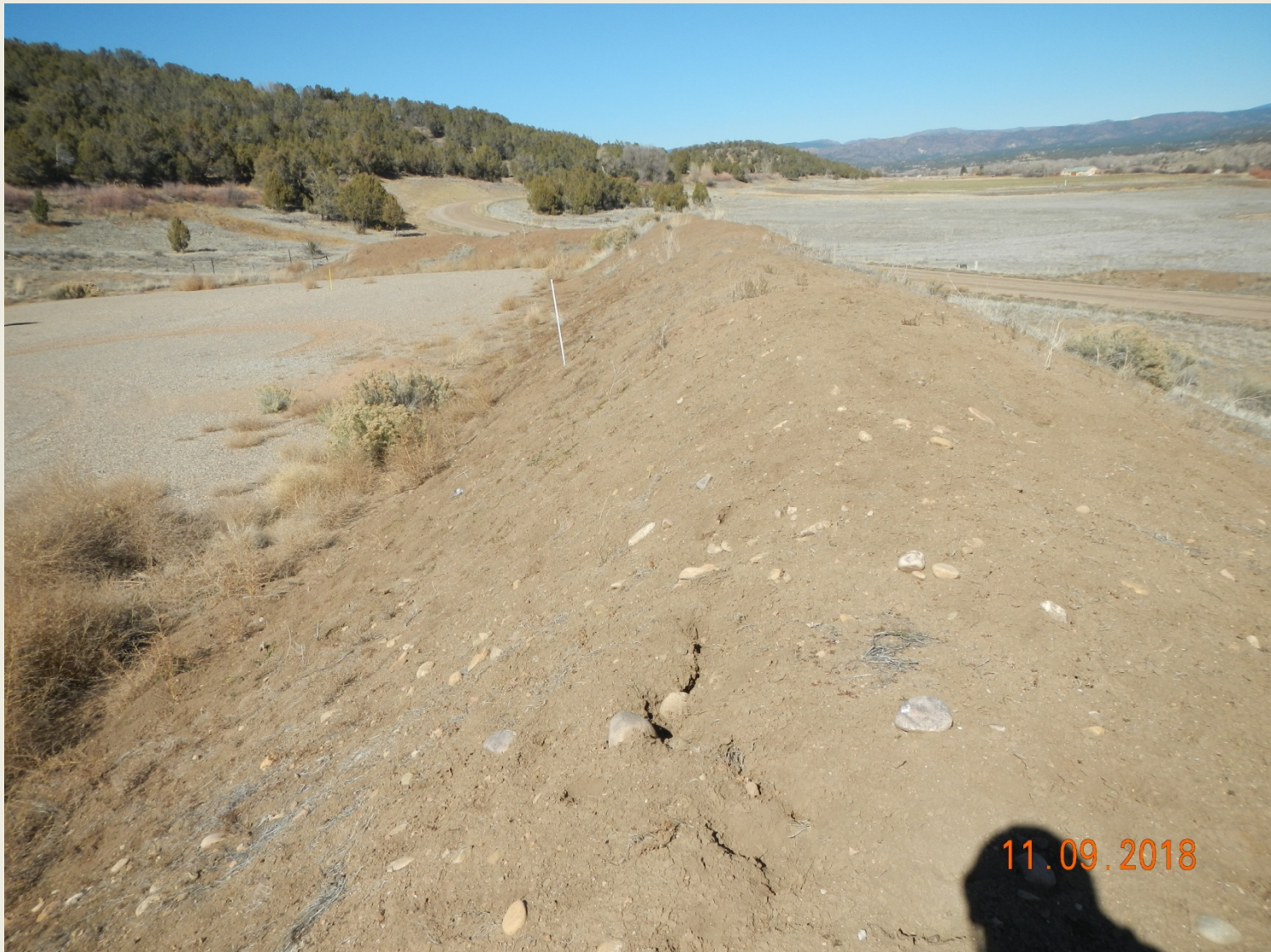
Photo 3. View of the eastern and northeastern berm (background), that needs to be stabilized with perennial vegetation, facing northward.
