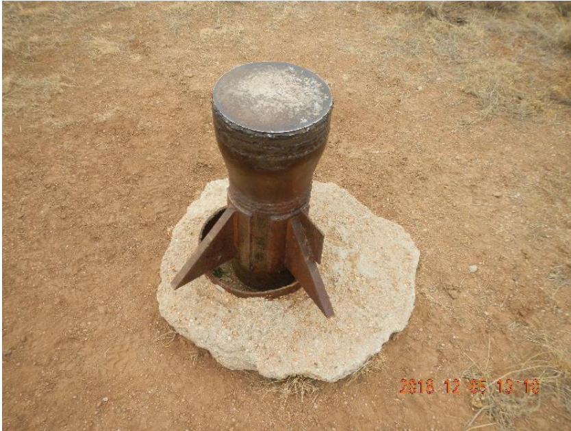
Photo 5: Close up of water/monitoring well.
