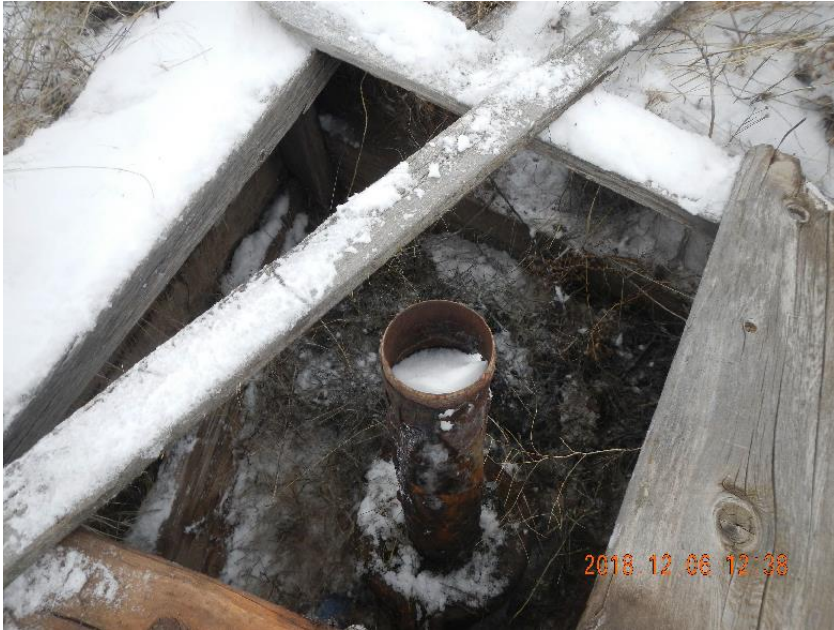
Photo 13: Casing with visible holes and frozed ice on side of casing.
