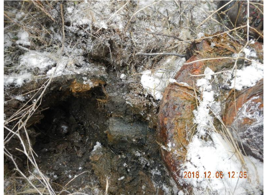
Photo 12: Bull plug on casing.
