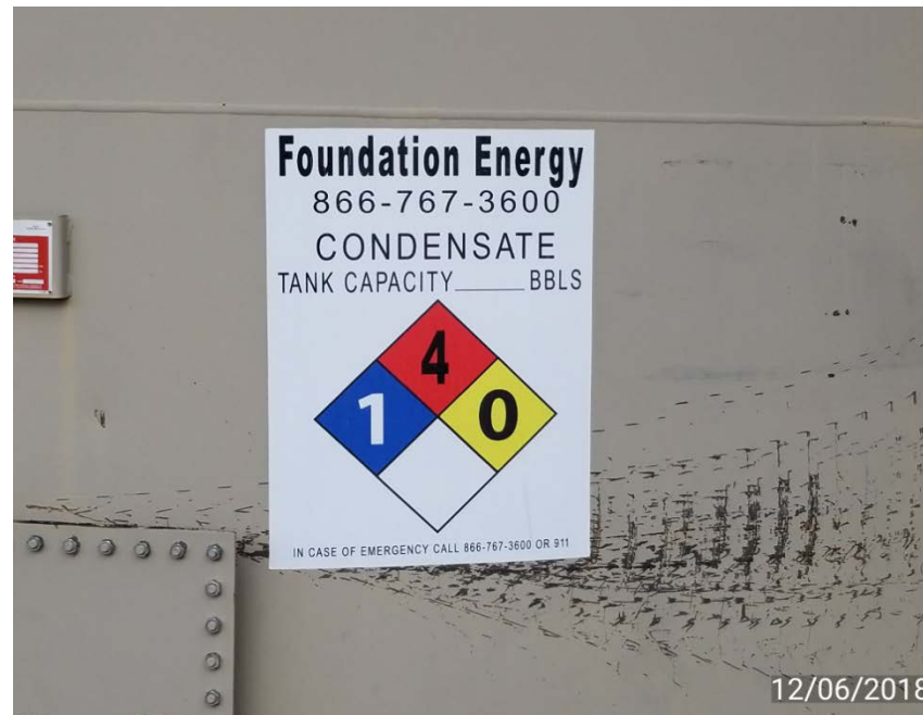
Photo 2. Tank sign missing capacity.
