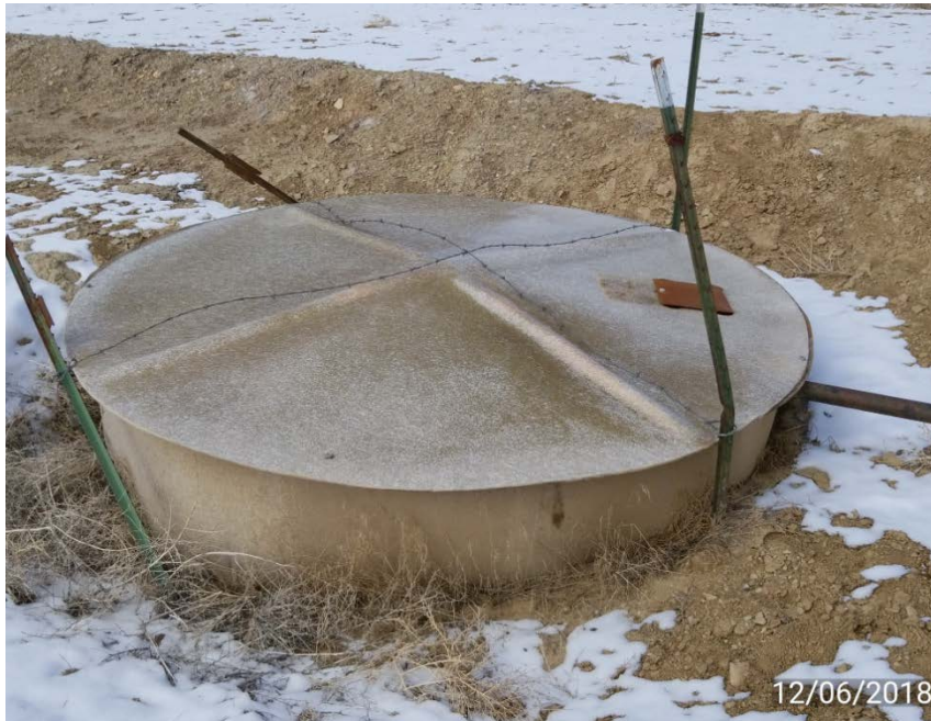
Photo 3. Buried tank without label.
