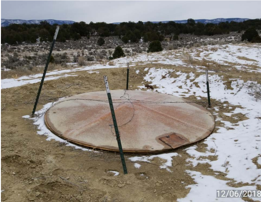
Photo 3. Buried tank without label.
