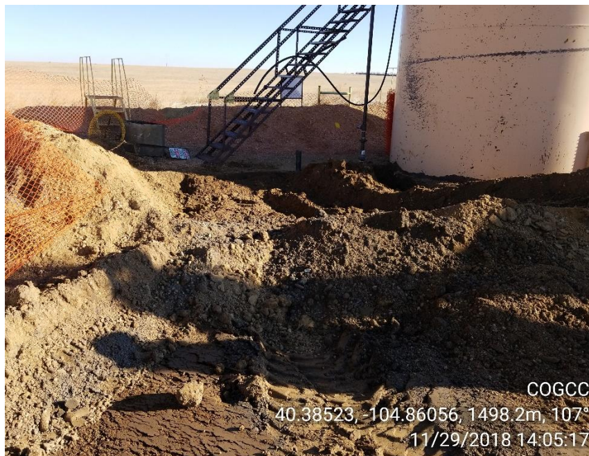
Photo 1 – Excavation area, partially backfilled after vault removal.
