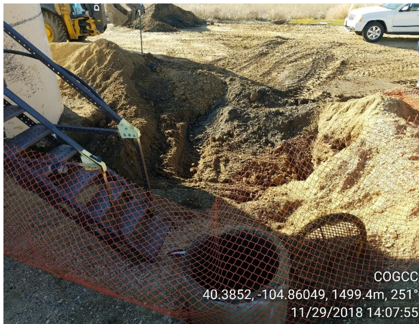
Photo 3 – Partially backfilled excavation area with impacted soils.
