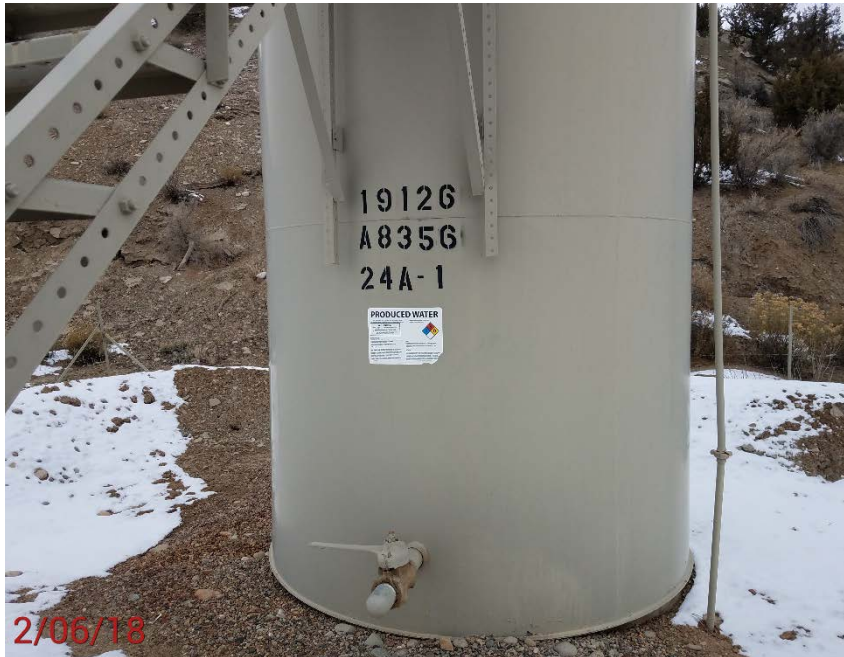
Location Photo #3, tank is missing barrel capacity.
