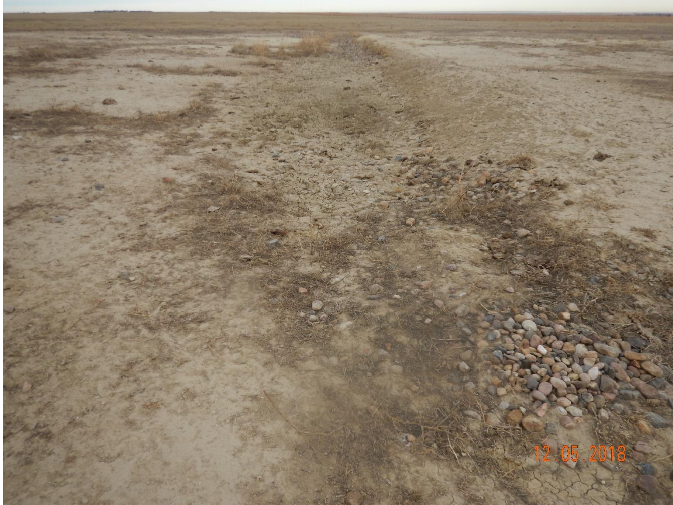
Photo 9: Photo taken from the south end of the disturbance area, facing east. Photo shows berm previously constructed for stormwater management.
