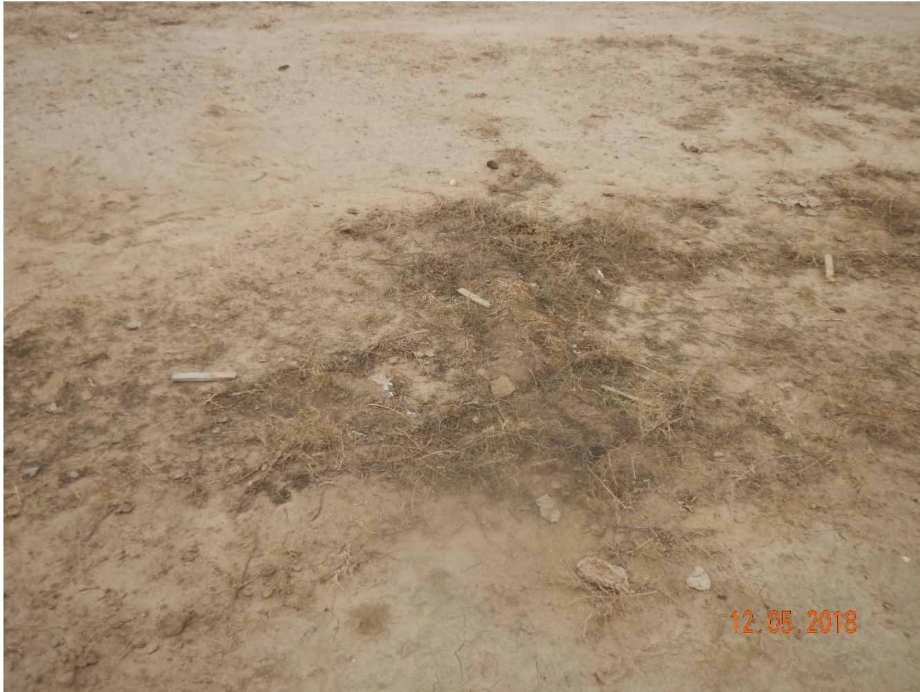
Photo 19: Photo taken from the north end of the location. Photo shows straw wattle BMP has been filled with sediment, is in disrepair, and no longer in proper functioning condition. Active stormwater monitoring and management does not appear to be ongoing.
