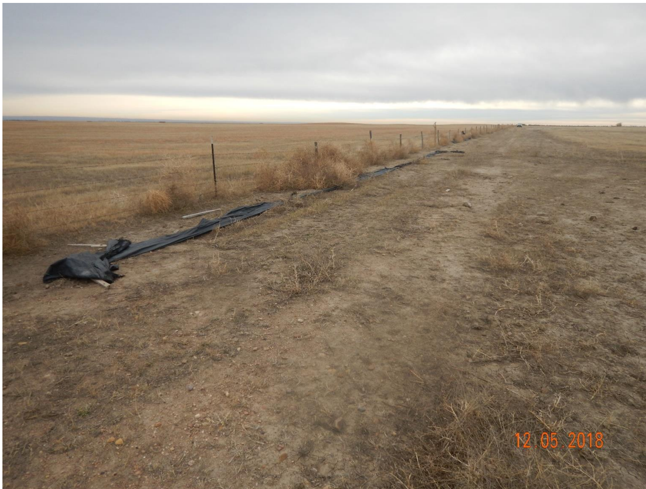
Photo 29: Photo taken from the east end of the location, facing south. Photo of silt fence. Previous inspections documented that areas of the silt fence in disrepair. Entire BMP is no longer in proper functioning condition.
