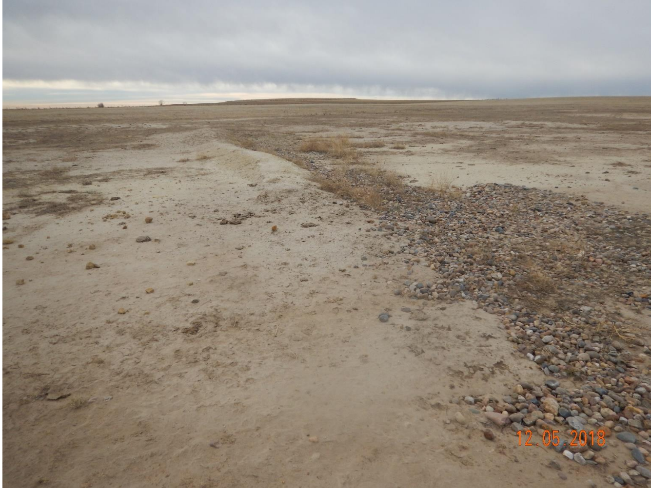
Photo 11: Photo taken from the north end of the southern berm, facing south. Photo shows berm previously constructed for stormwater management.
