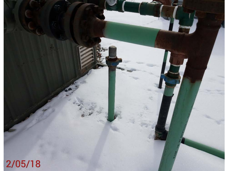
Location Photo #4, unmarked flow line riser near meter run.
