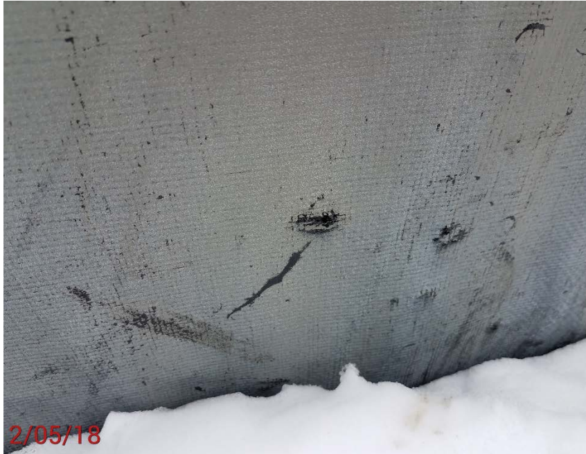
Location Photo #7, Small holes in battery liner.
