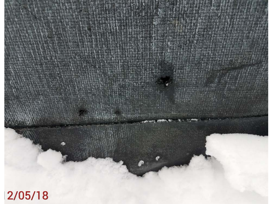
Location Photo #10, Small holes in battery liner.
