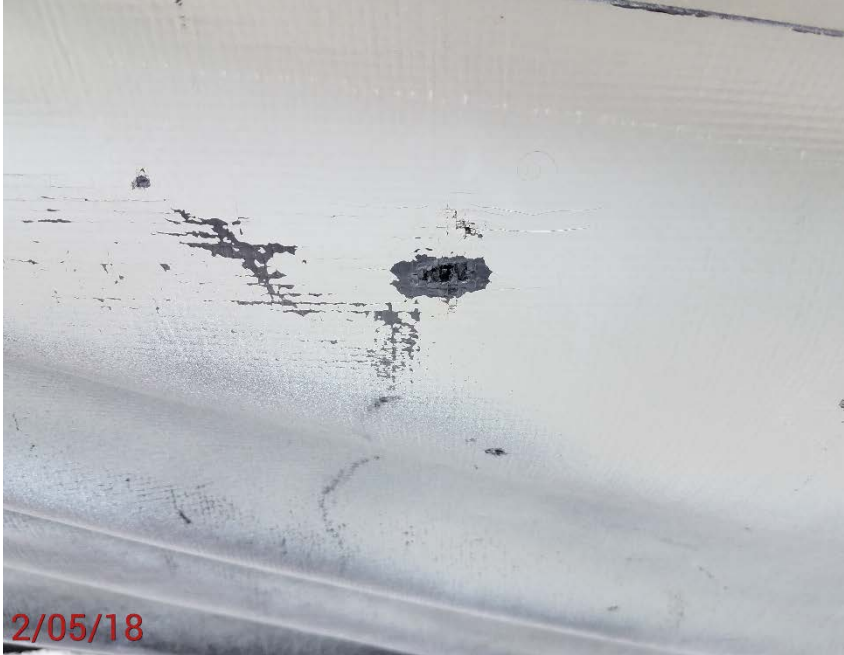
Location Photo #9, Small holes in battery liner.
