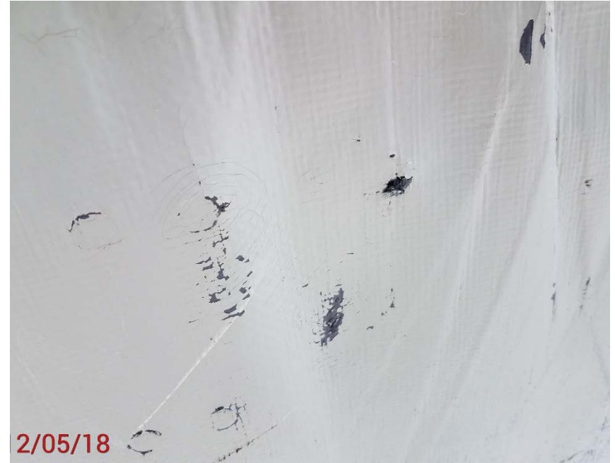
Location Photo #8, , Small holes in battery liner.
