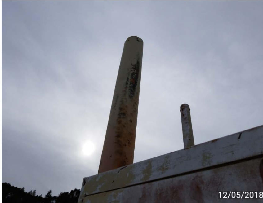
Photo 3. Separator stack without bird protector.
