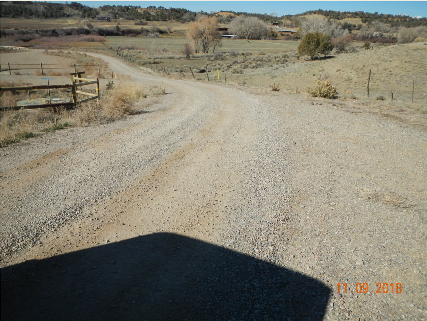
Photo 5. View of road surface maintained in good repair.
