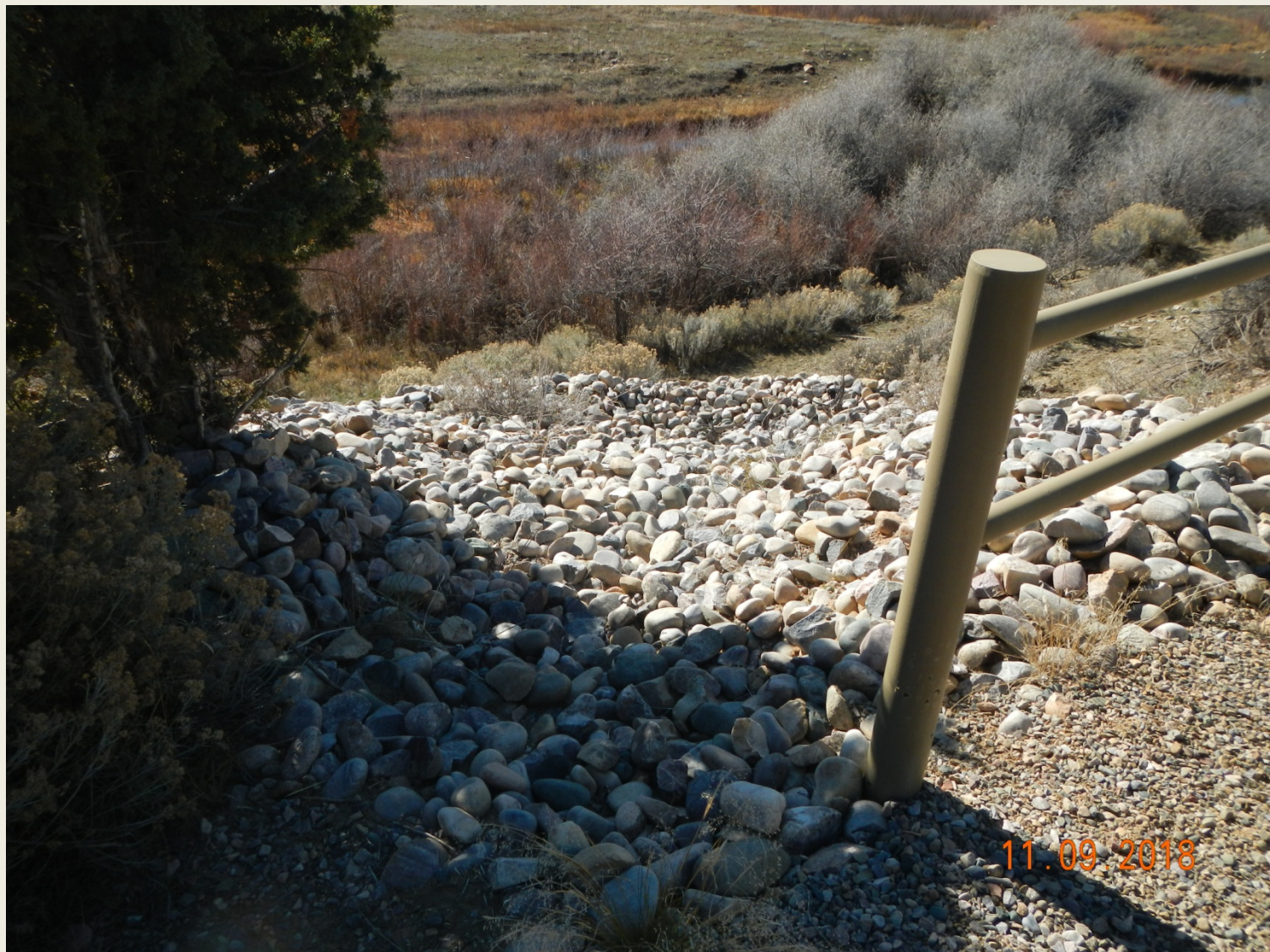
Photo 3. View of cobble run-down in the northeastern project area that appears to be functioning.
