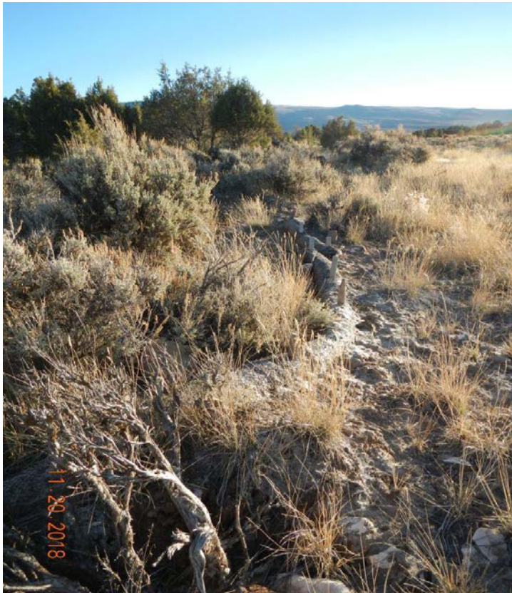
Photo#4: Wattles are installed on East perimeter.
