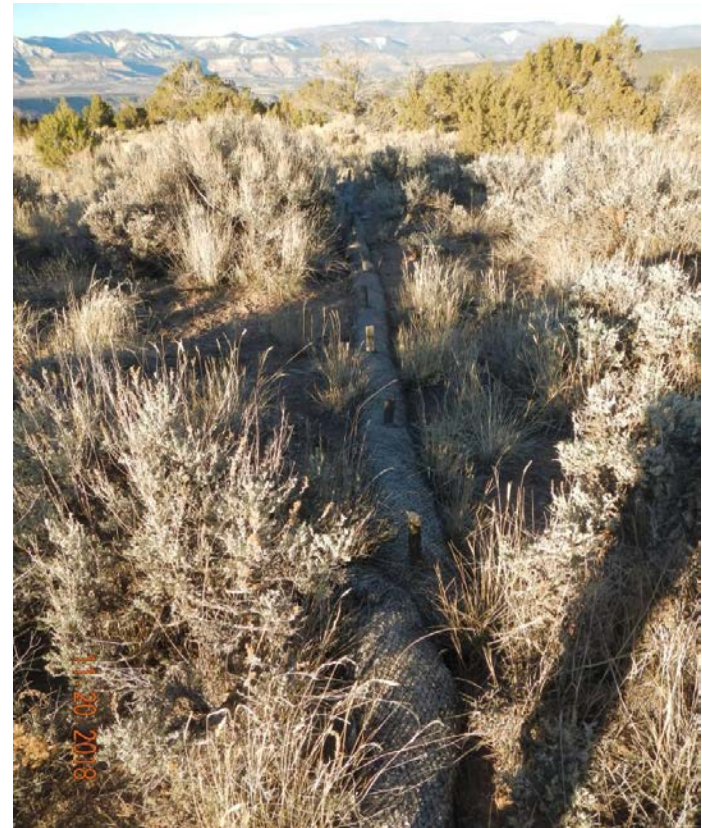
Photo#5: Wattles are installed on East perimeter.
